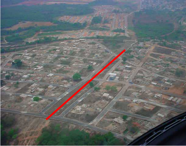
Figure 3.2 – Encroachment around the pipeline right-of-way.
