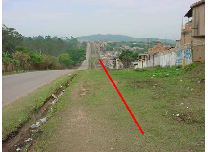
Figure 3.4 – Encroachment around the pipeline right-of-way.
