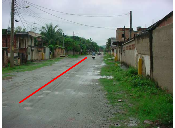
Figure 3.5 – Encroachment around the pipeline right-of-way.
