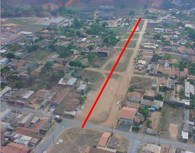
Figure 3.3 – Encroachment around the pipeline right-of-way.
