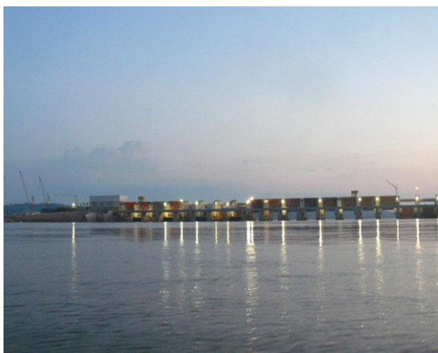
Figure 10 – Jirau Hydroelectric Power Plant, Madeira River/state of Rondônia (Photo: Daniely Félix-Silva).
